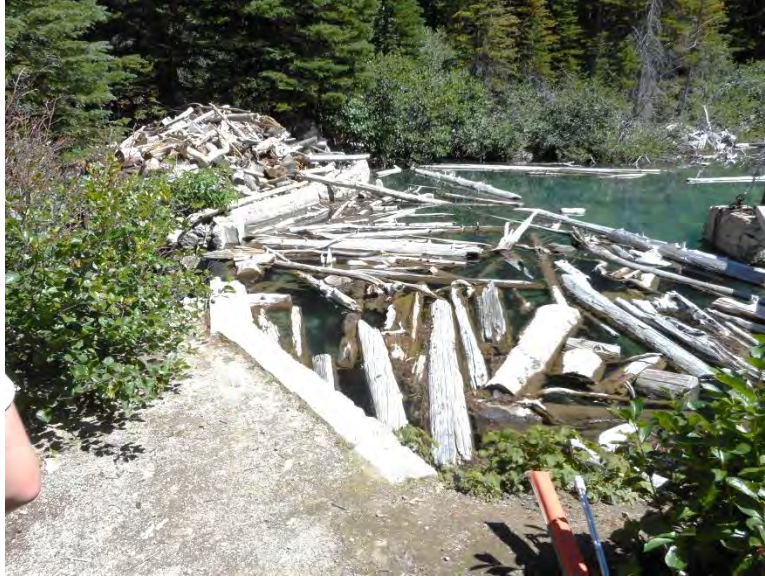
Photo 22 - Colchuck Lake Dam, View from West Abutment
