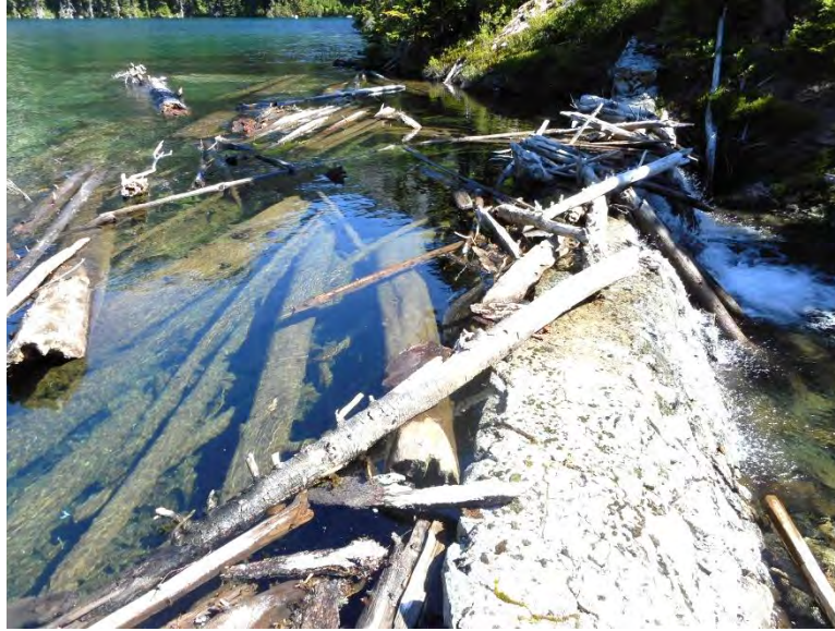
Photo 7 - Square Lake Dam along Crest
