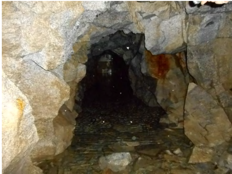
Photo 4 - Square Lake Inside Outlet Works Tunnel (Gate Visible)
