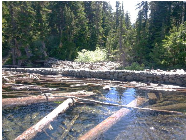
Photo 6 - Square Lake Dam and Spillway (From Lake)
