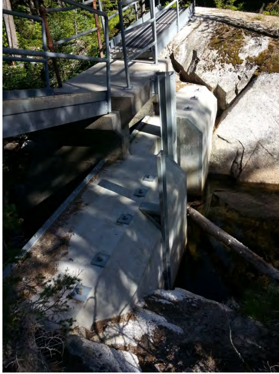
Photo 37 - Nada Lake Dam (Recently Reconstructed by USFW)
