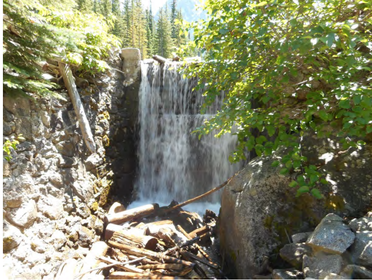
Photo 24 - Colchuck Lake Spillway
