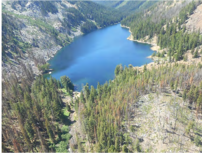
Photo 17 - Eightmile Lake Dam - Aerial View
