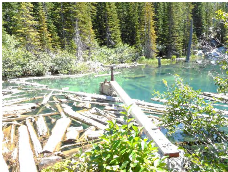
Photo 18 - Colchuck Lake Gate Actuator and Tower
