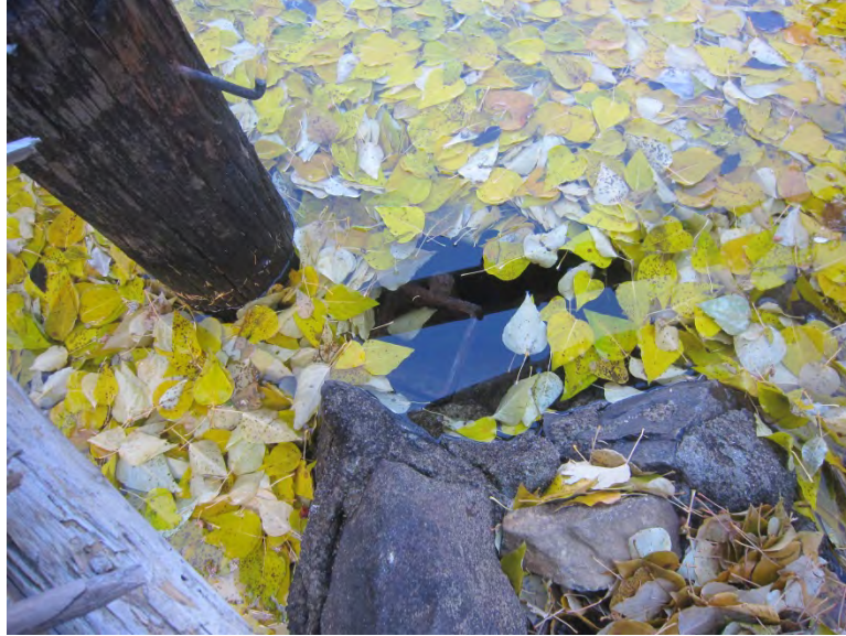
Photo 16 – Submerged Gate Location
