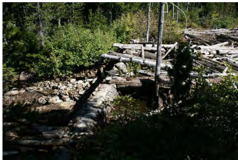
Photo 28 - Lower Snow Lake Dam, View from Lower Snow Lake Side
