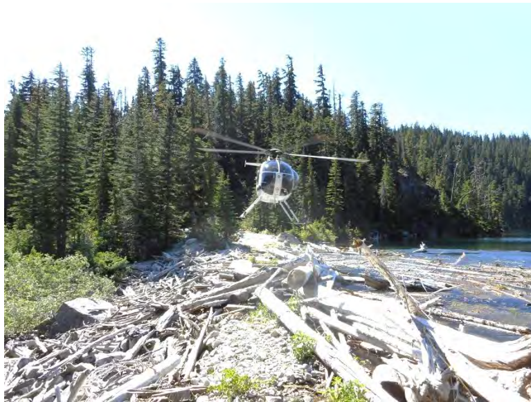
Photo 13 – Lower Klon aqua Dam Embankment, View along Crest from North
