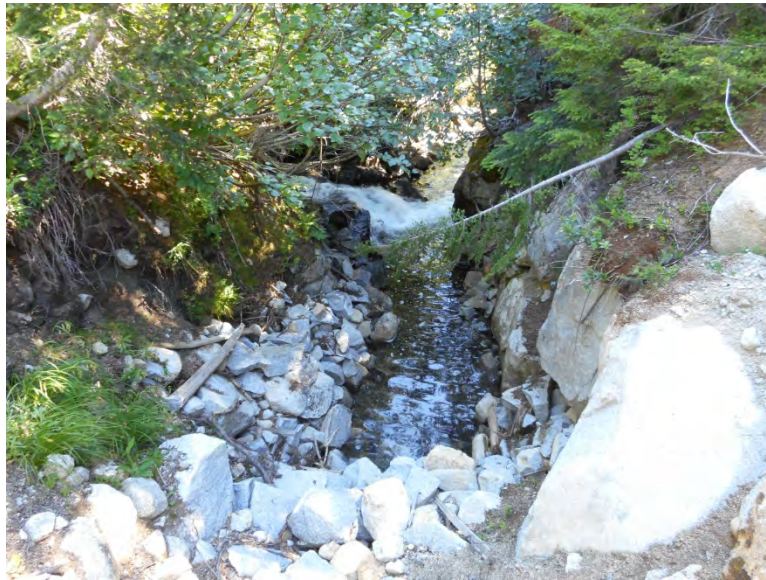
Photo 11 – Lower Klonaqua Outlet Works Channel (No Flow, Backwater Present)
