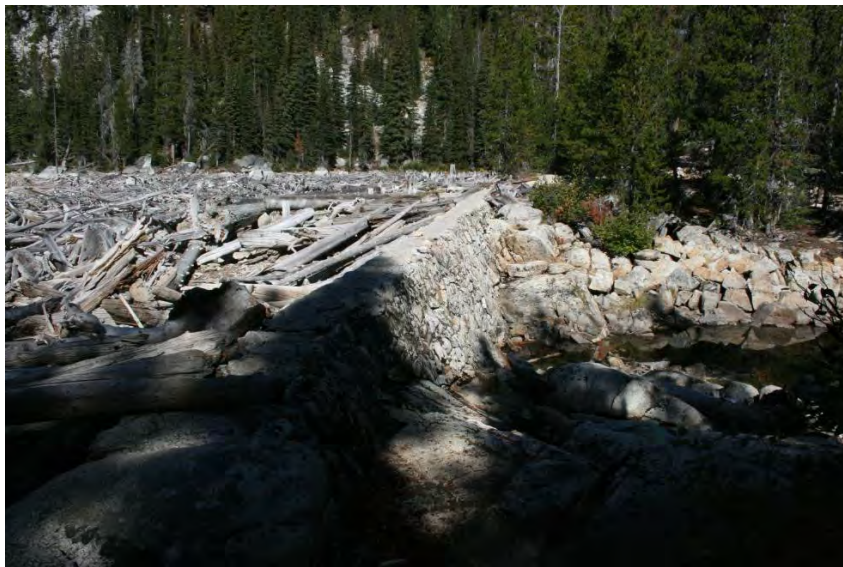
Photo 26 - Upper Snow Lake Dam and Spillway
