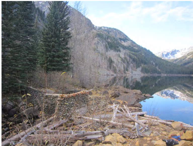
Photo 14 - Eightmile Lake Dam (Submerged Gate Not Visible)
